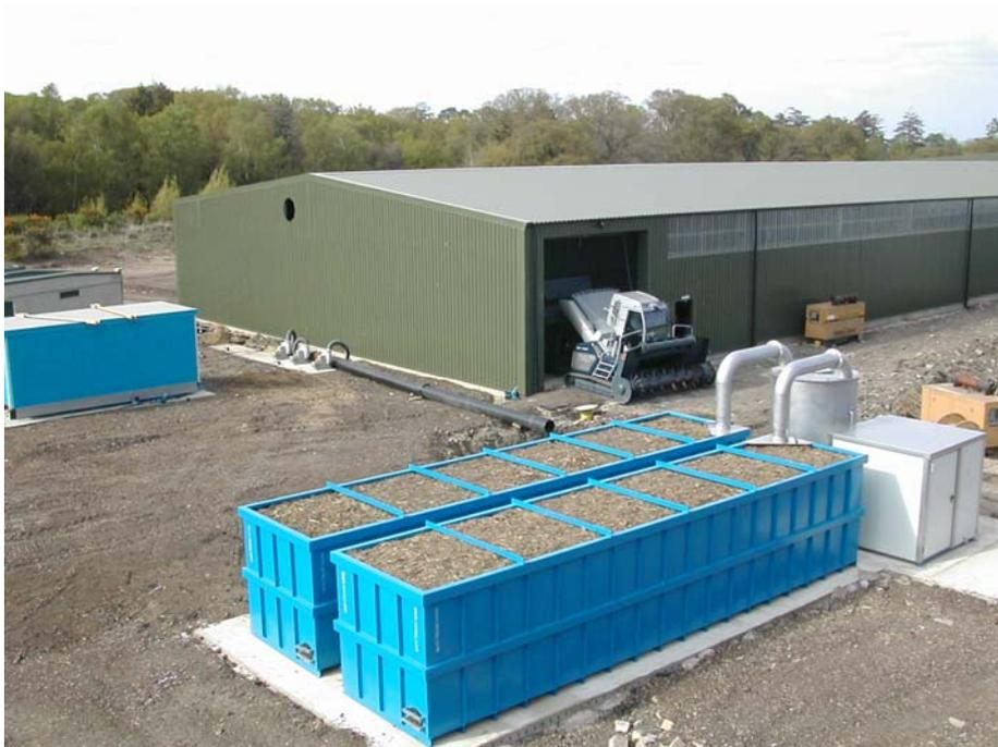
**Plate 1 New Earth Technology showing biofilter and scrubber in foreground and composting hall in the background with the windrow turner emerging from the hall.**
